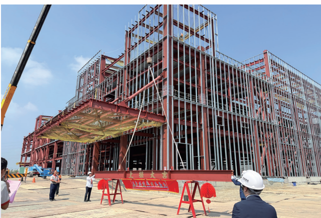
2025.10.16 Beam-raising ceremony for Ebara Precision Machinery Taiwan's second factory in Tainan
