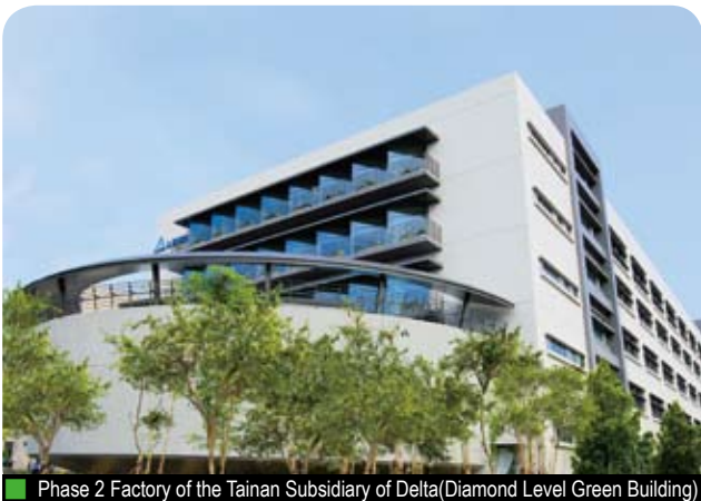
Phase 2 Factory of the Tainan Subsidiary of Delta(Diamond Level Green Building)
