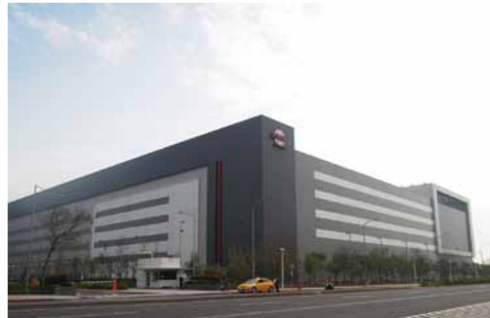
STSP's Green Building – TSMC's P4 Building for Fab 14 Received Taiwan's EEWB Diamond Green Building Certification (September 3, 2012)
