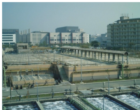
Phase II of the Wastewater Treatment Plant in the TSP
