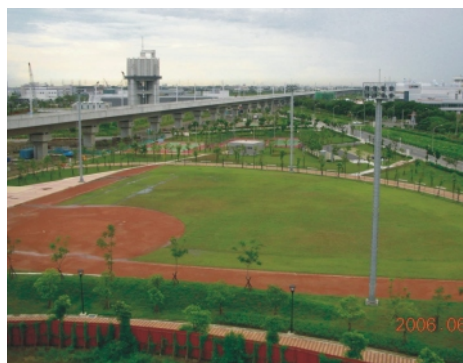
Softball Pitch, One of the Outdoor Facilities of the Sports Park
