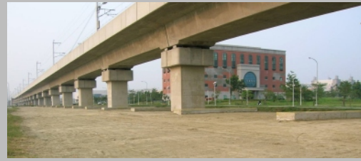
The Site after Completion of the Reinforced Structure Construction (An Underground Framed Structure Constructed between the Piers of the Taiwan High Speed Rail. The Protuberances on the Ground are the Vibration Damper Maintenance Holes.)
