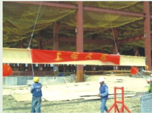
Beam Construction of Allied Material Technology (October 10)
