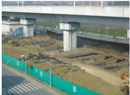
Construction of Foundation Reinforcement
