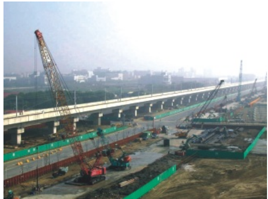
Construction of Elastic Vibration Reduction Wall
