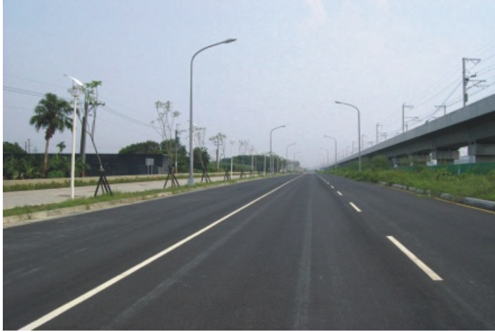
Residential Area in the Northern Side and East 1 and 2 Area Development Project (Roads of East 2 Area )
